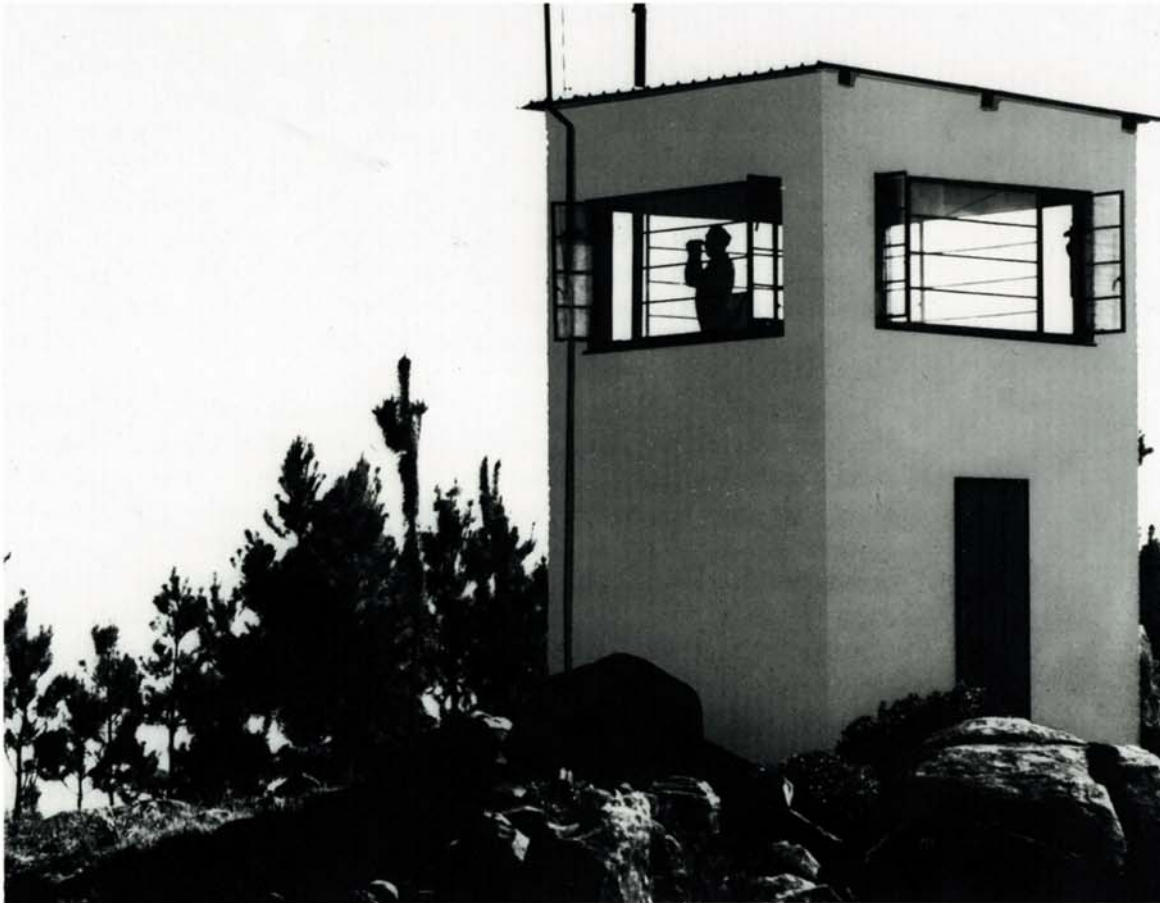
Early firewatch tower in the Eastern Transvaal.
