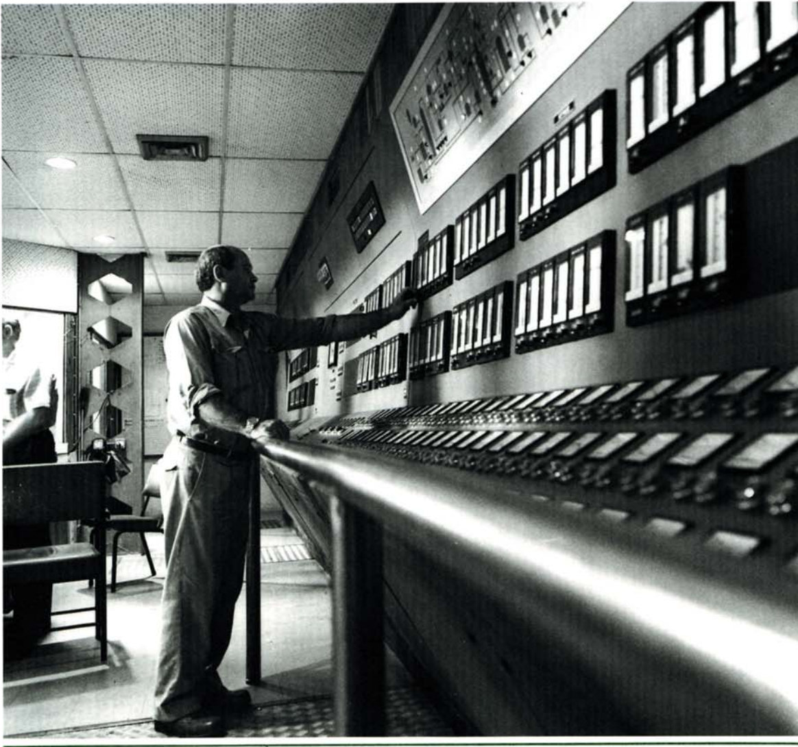
Control room serving Enstra's bleaching plant.
