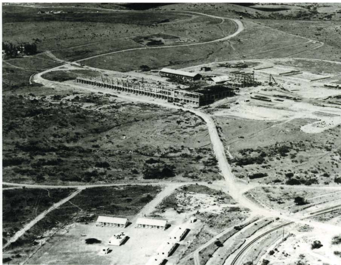
Tugela mill under construction, photographed in 1952.
