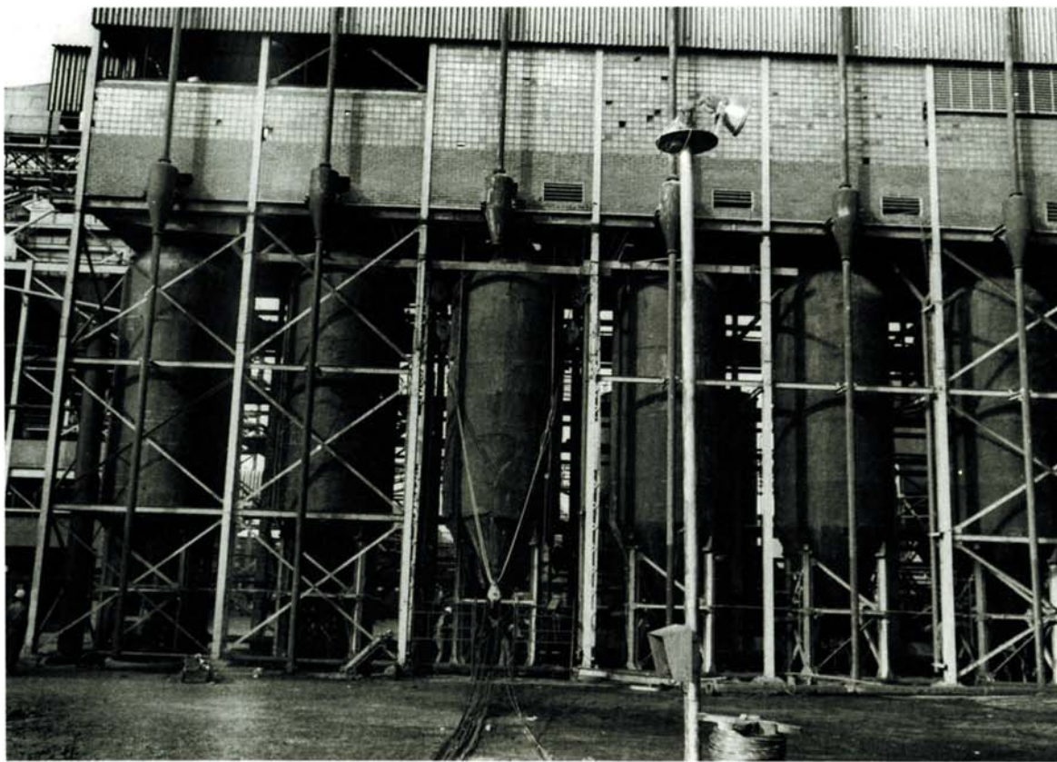
Batch digesters at Tugela, to be replaced by a continuous digester.
