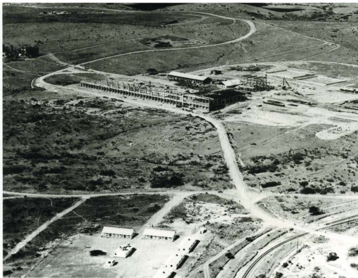
Tugela mill under construction, photographed in 1952.
