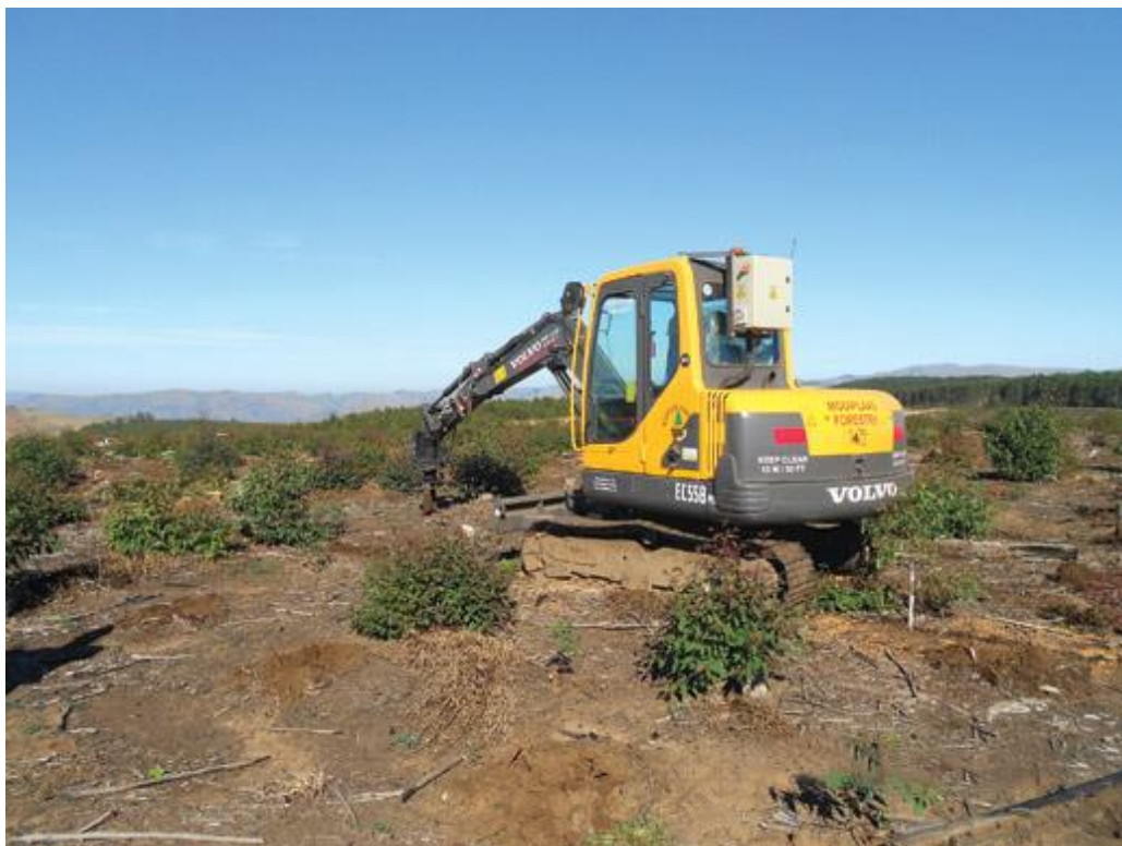
Photo 4: A compact excavator with a head attachment. 6
