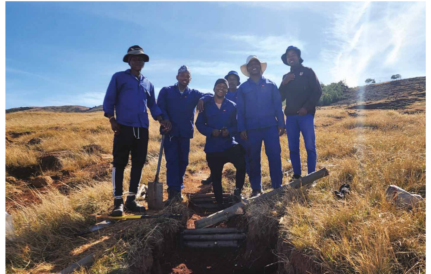
Alien vegetation clearing and water catchment management initiatives in collaboration with the Institute for Natural Resources, have provided employment opportunities to the people of Nzinga and Qutshini.
