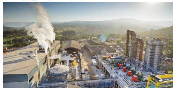
Approximately 20,000 tons of chips generated from the logs are sold to Ngodwana Mill for use in their boilers.
